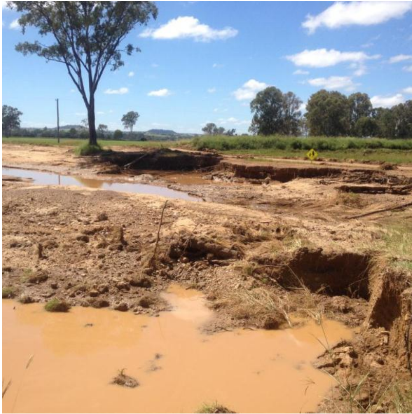
Scouring in paddocks from Hurdle Gully Outfall
