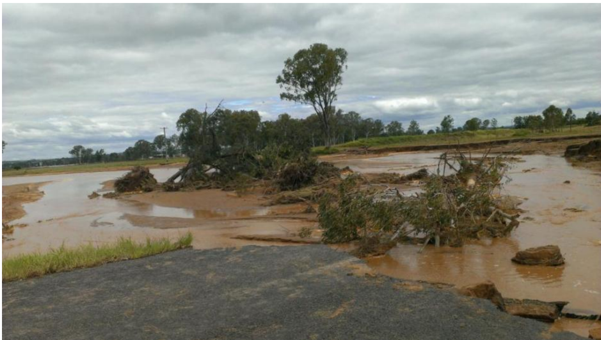
Airport Drive, Dowlings Flood Damage from Hurdle Gully (hole approx. 2 metres deep). This is a Flood Recovery project that was about to commence, due for completion in May 2015.
