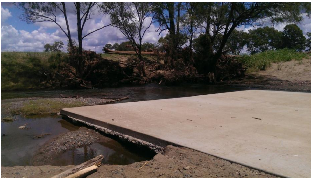
Creek crossing project finished in late 2014 damaged by TC Marcia flooding event and in need of repair
