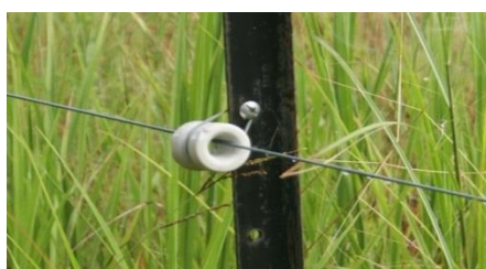
Steel post porcelain insulator: attached with a 6 mm bolt and nylock nut.
