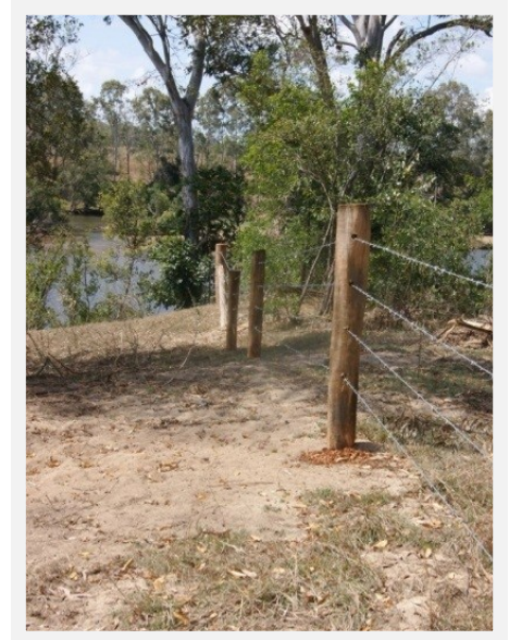
Fence erected to prevent cattle entering the gully and causing erosion
