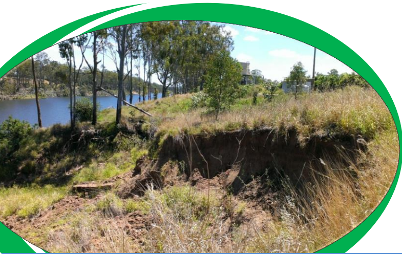
Riverbank erosion resulting from the floods
